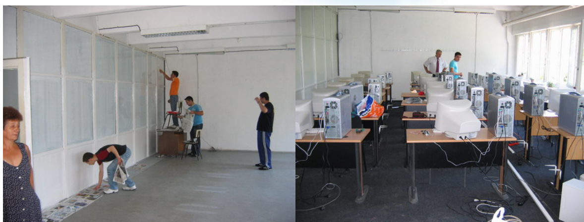
Arranging the centre – installing equipment, cables, etc.
